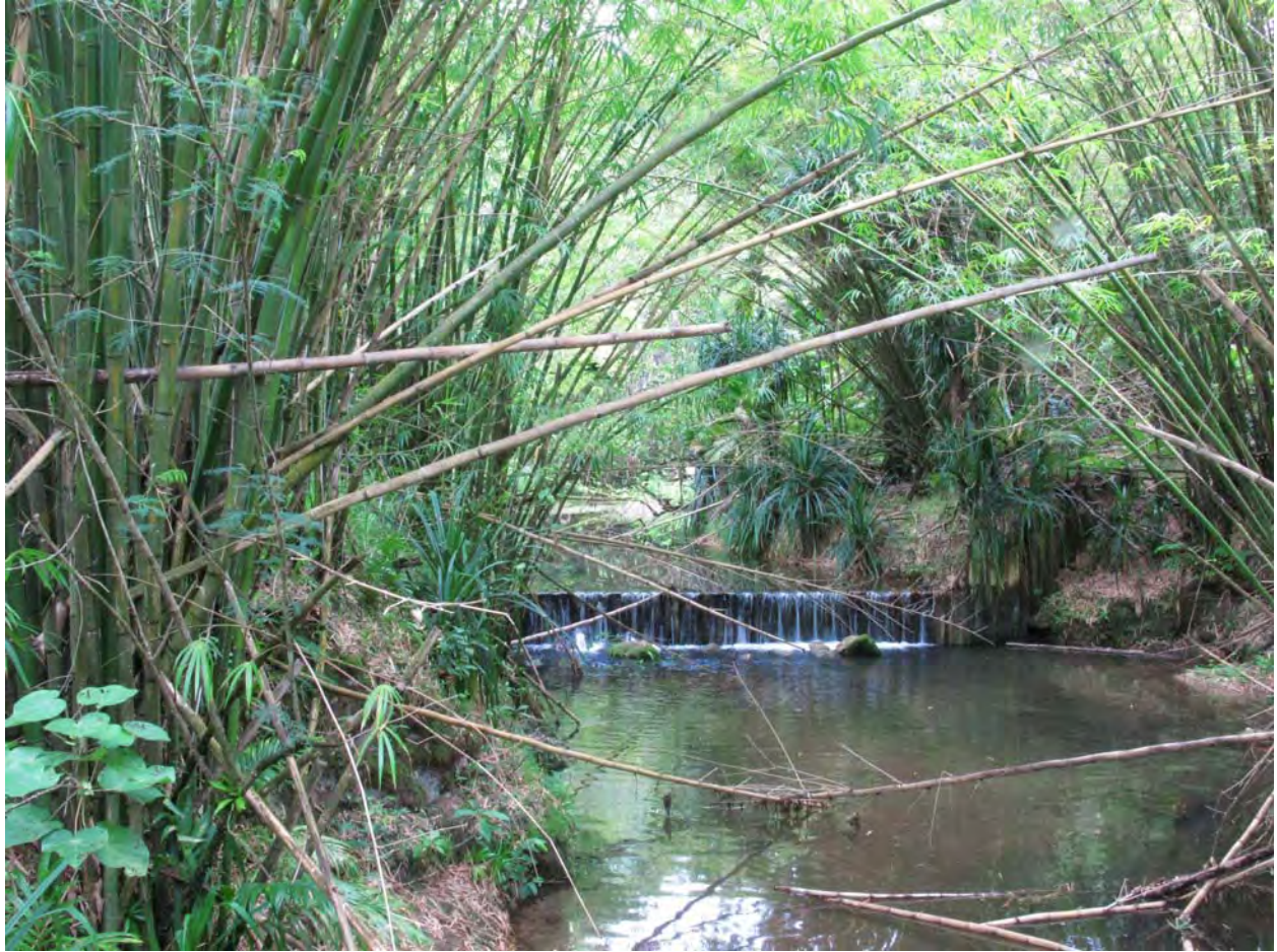
Text Figure 1817-7. An upstream view of the Tolaeyuus River from the bridge, showing a low sheet-piling dam. Such a dam could theoretically raise the water level within the underground aquifer, and thus increase its storage capacity to maintain supply during low-flow dry season periods. Patches of bamboo (foreground) and small Pandanus tectorius (background in vicinity of the sheet-piling dam) are quite common on both sides of the river along Transect 1 on the left and Transect 2 on the right.
